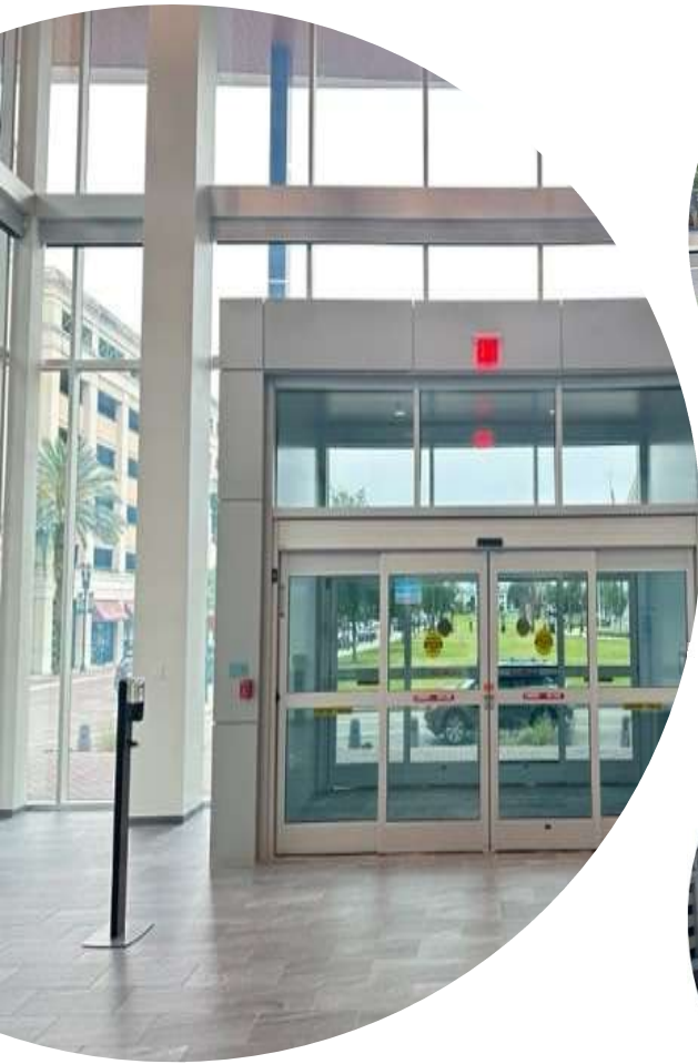
Pearl Street Exit
