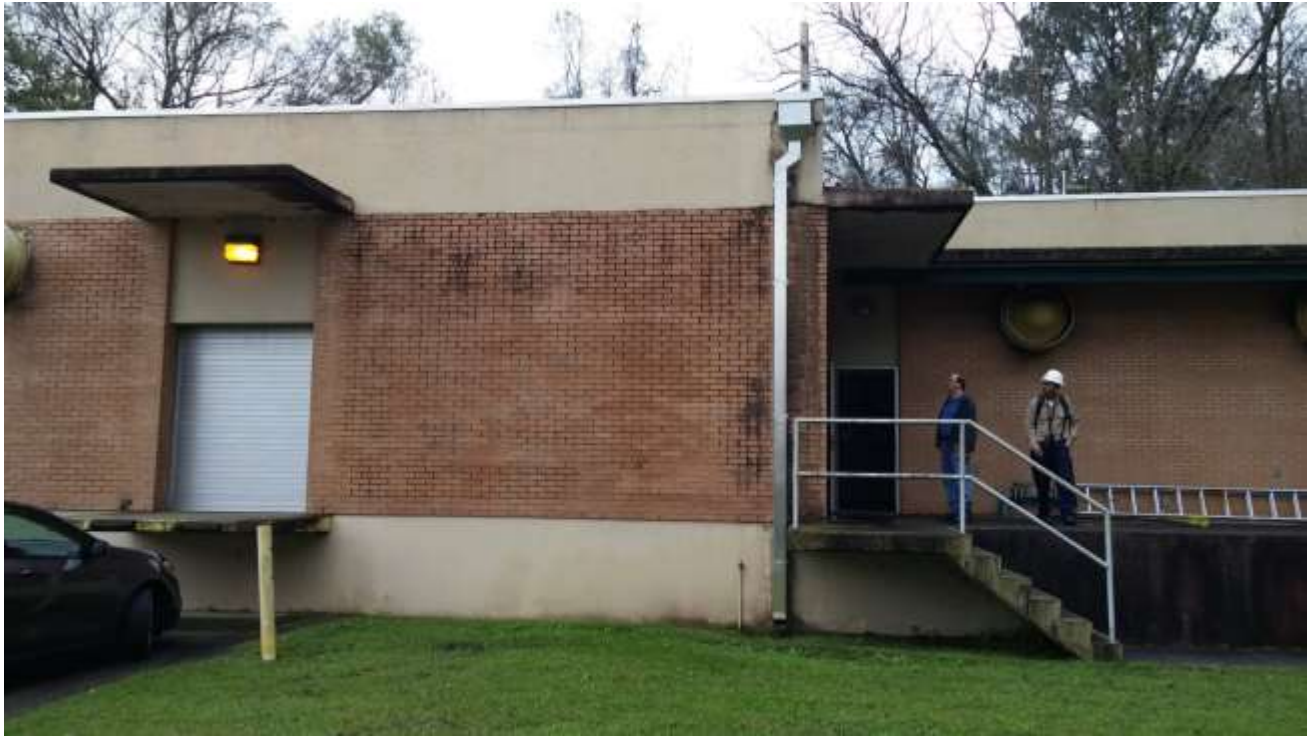
Big Wilson PS – North Part of the Building
