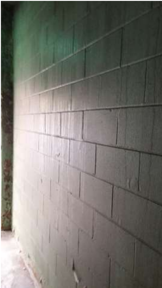
Photos 9 and 10 – Paint peeling from the Screen Room Walls
