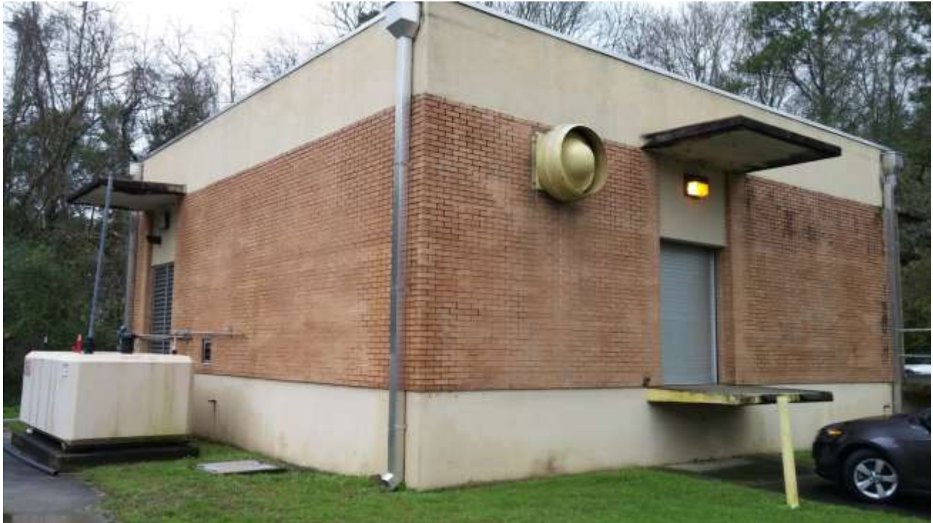
Big Wilson PS – Northeast Part of the Building
