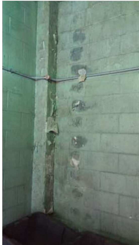
Photos 9 and 10 – Paint peeling from the Screen Room Walls
