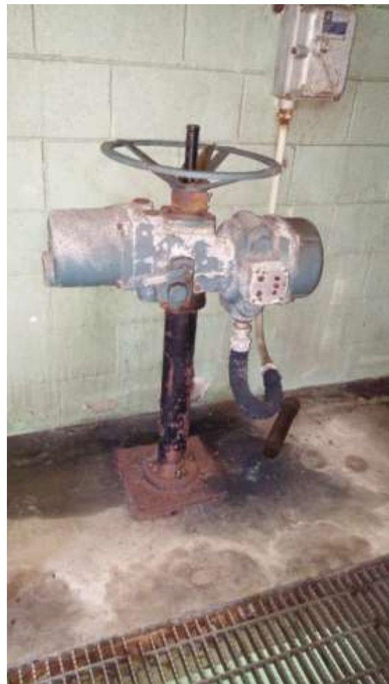
Photo 6 & 7 – Frozen Sluice Gates and Actuators
