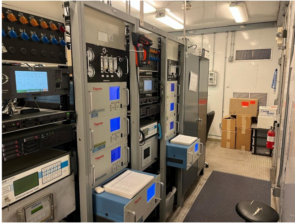
Figure 1: NS 1 and NS 2 CEMS Analyzers
