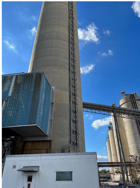
Figure 4: N03 Stack with Umbilical Tray
