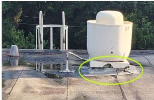
Curb on exhaust fan to be raised to 8" above new finished roof by installing necessary 2x4 treated lumber and install new flashing. Exhaust fan at the corner to be liquid flashed and pocket removed.
