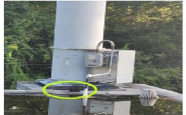
Curb on exhaust fan to be raised to 8" above new finished roof by installing necessary 2x4 treated lumber and install new flashing. Exhaust fan at the corner to be liquid flashed and pocket removed.
