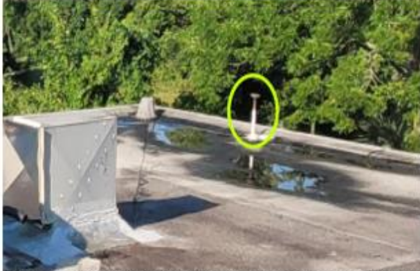
Remove conduits and pitch pockets, pull pipe through roof or cut flush with deck, and then cover openings, see four photos above.
