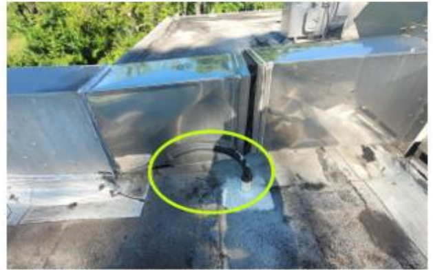
Remove conduits and pitch pockets, pull pipe through roof or cut flush with deck, and then cover openings, see four photos above.
