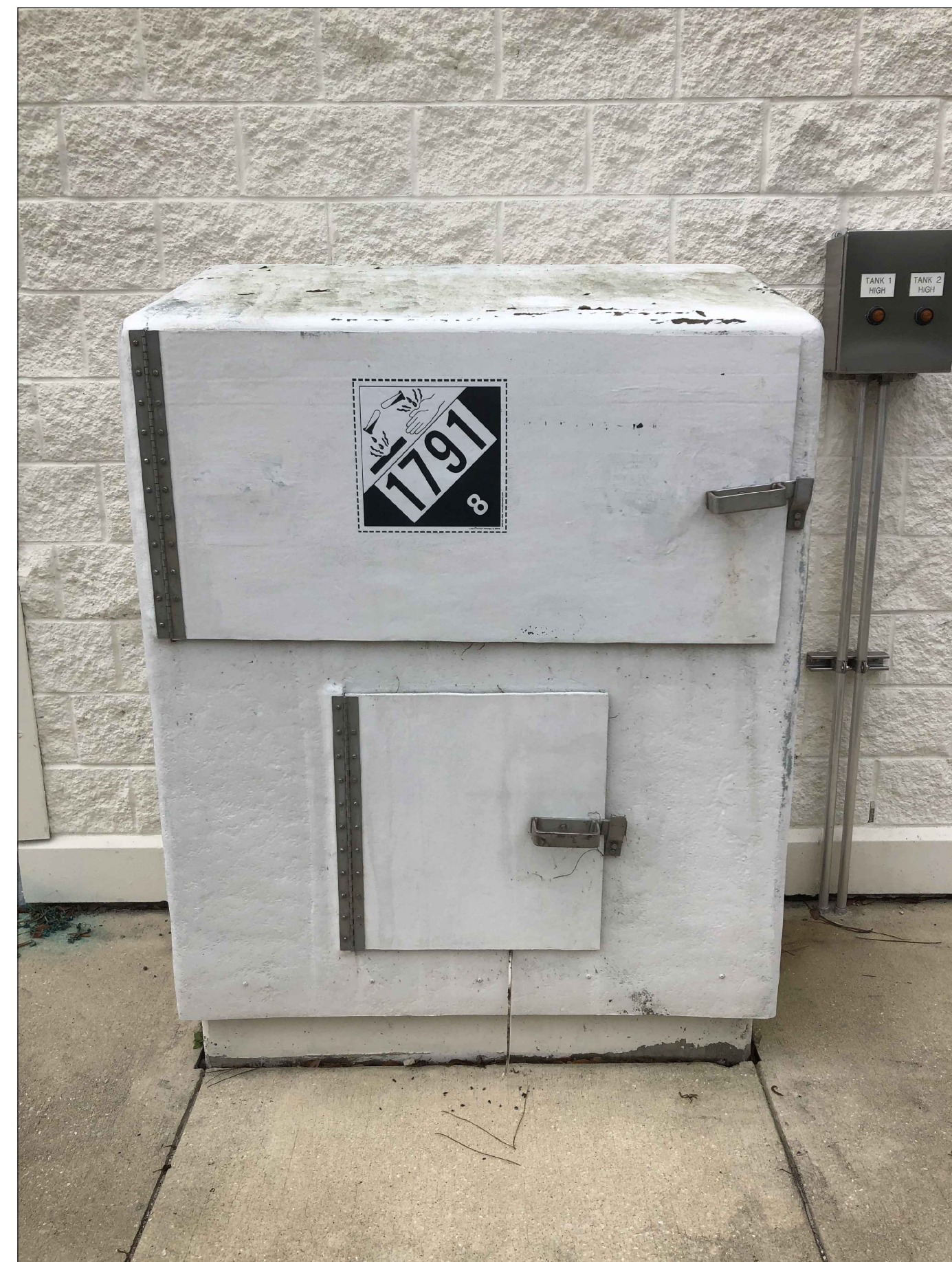
CHEMICAL FILL STATION NTS
