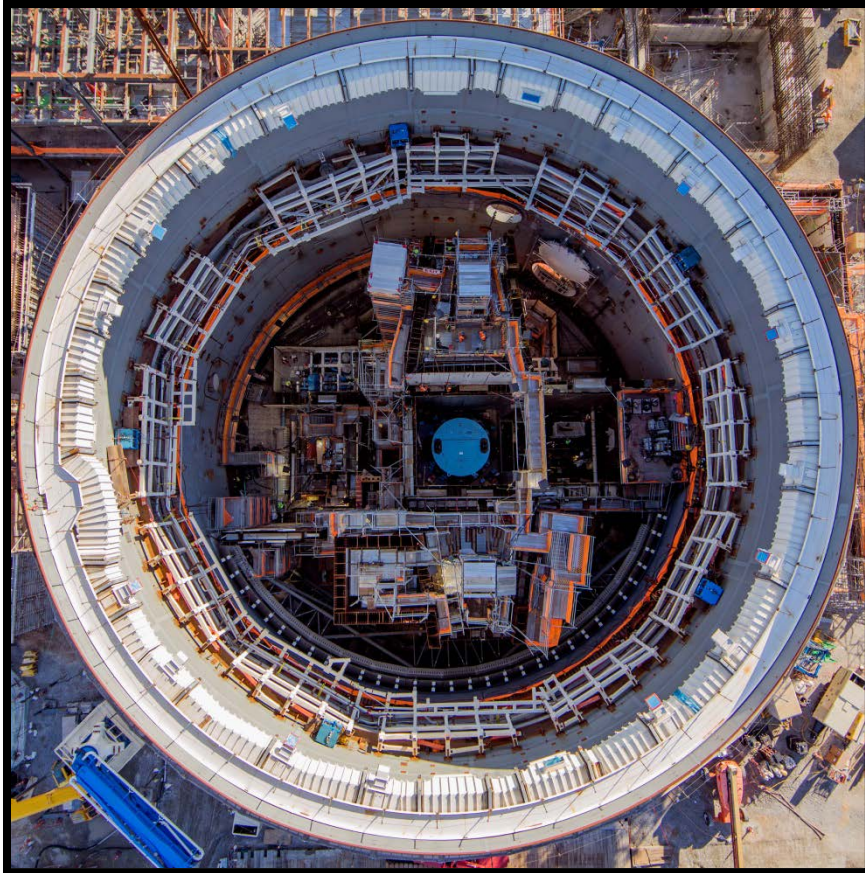
Inside Unit 3 Containment
