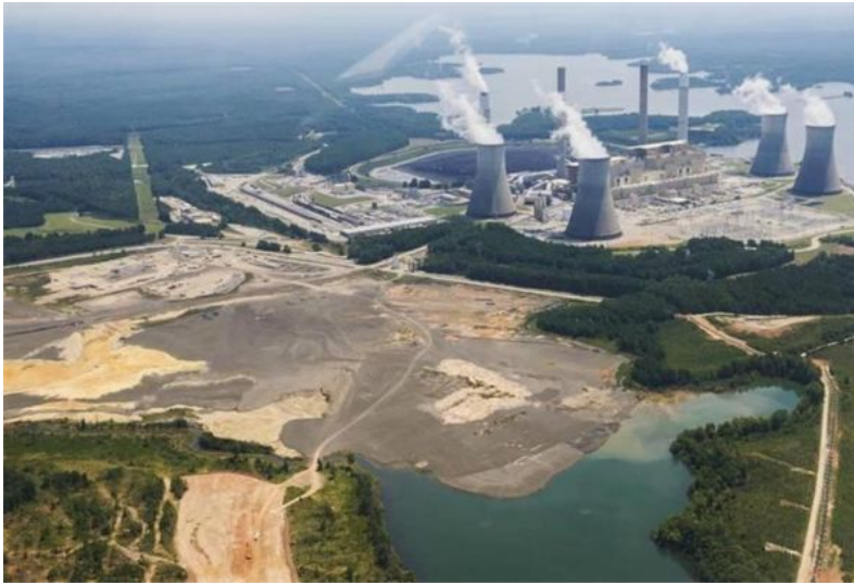
Plant Scherer. Ash Pond in Foreground
