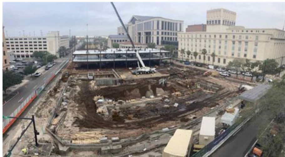
West facing view of office building construction
