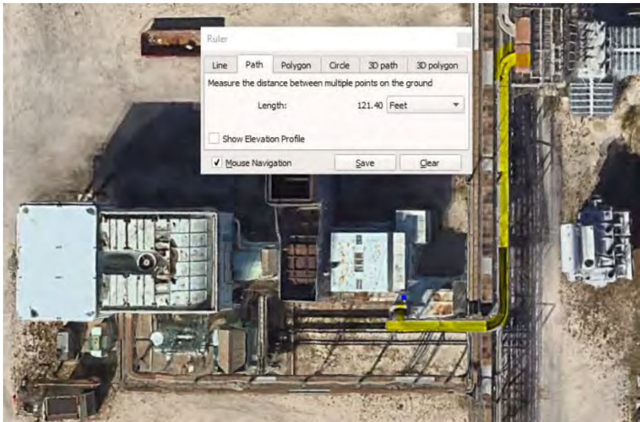
Cable Tray visible on Google Earth.
