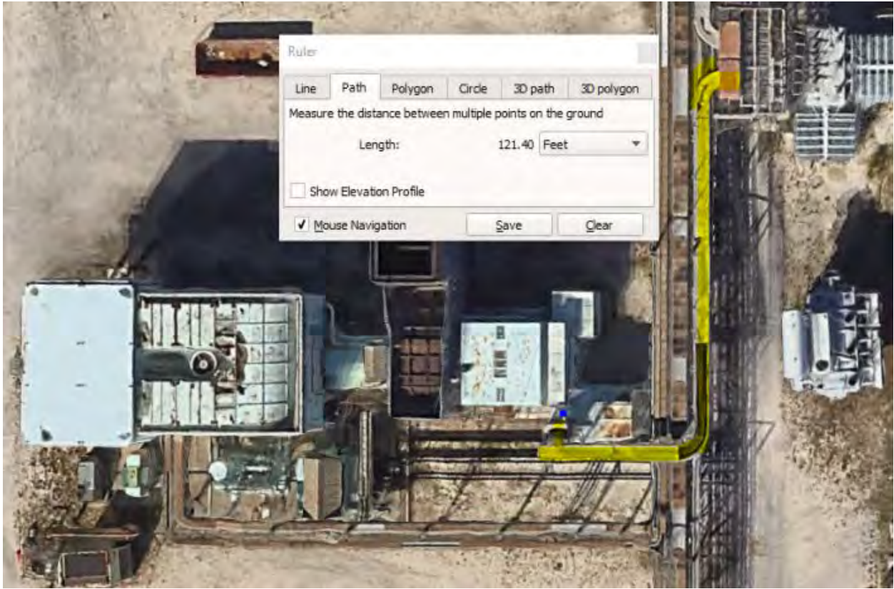
Cable Tray visible on Google Earth.
