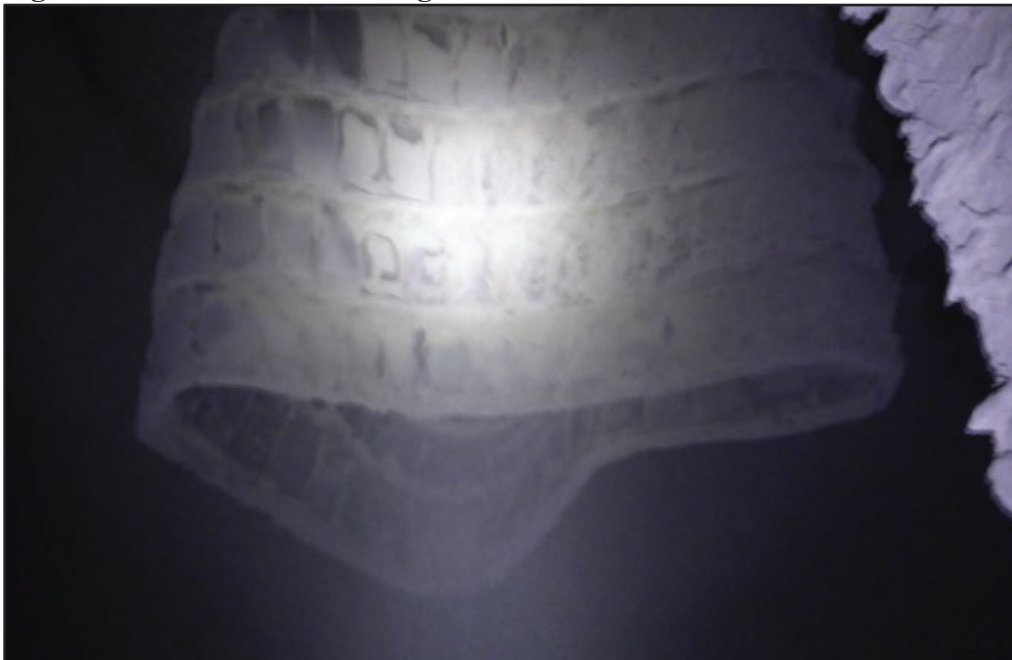
Figure 3. Vortex Finder Damage
